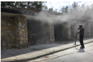
Curbed entrance being cut out.
