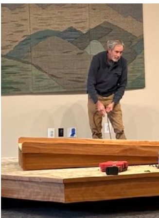
Doug Installs New Cable
