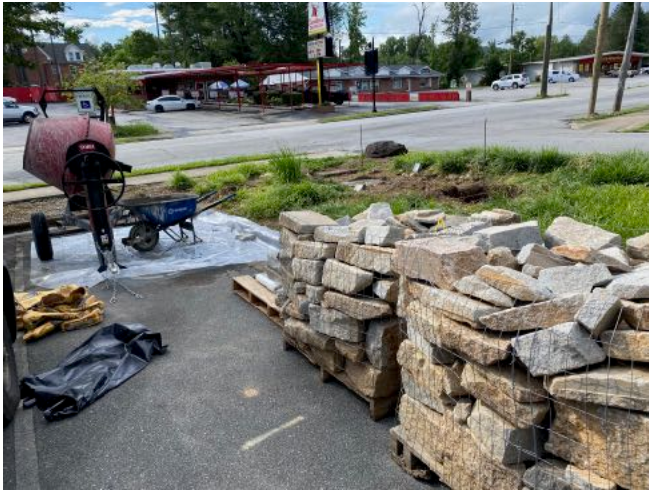
Work on the new sign moved forward in earnest this week, with footings excavated, rebar laid, concrete poured and columns built with a channel for electricity. Stone work begins today (Friday).
