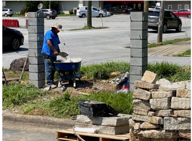
Work on the new sign moved forward in earnest this week, with footings excavated, rebar laid, concrete poured and columns built with a channel for electricity. Stone work begins today (Friday).
